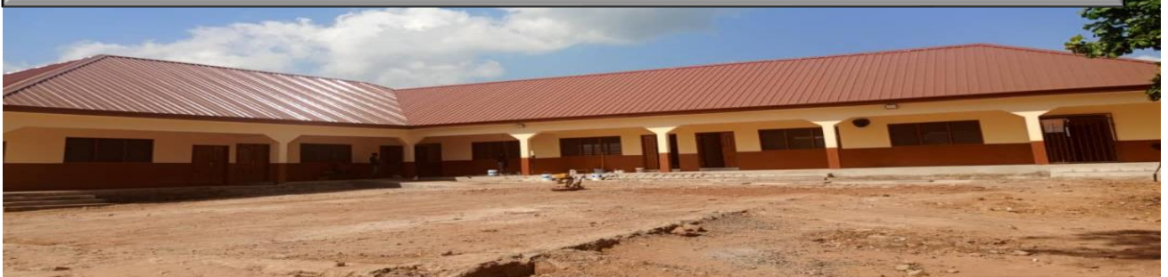
3-unit classroom block with 6-seater toilet facility, a library and an Ultra-modern ICT laboratory in Somanya Methodist school By Hans Djaba
