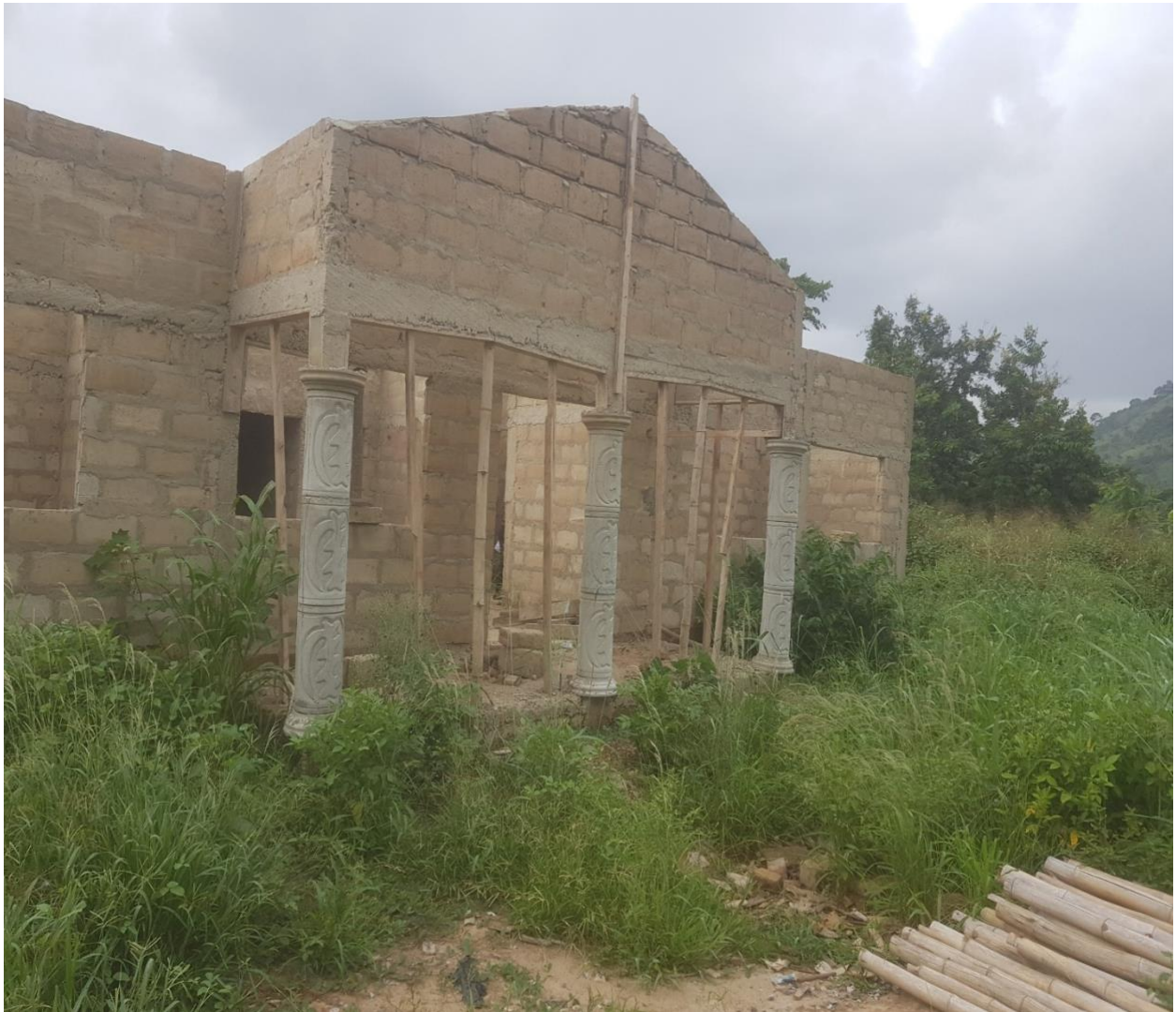
CONSTRUCTION OF POLICE POST AT AGOGO - DACF (52% COMPLETED)
